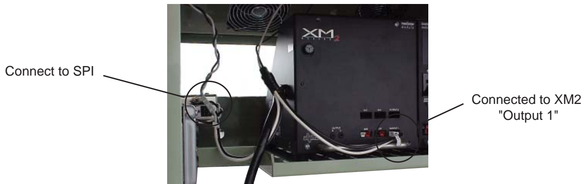
Fig. 5-14, Cooling Fan Plugged into Power Supply and SPI
